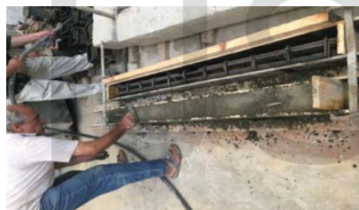
Fig (29): Beams during pouring
